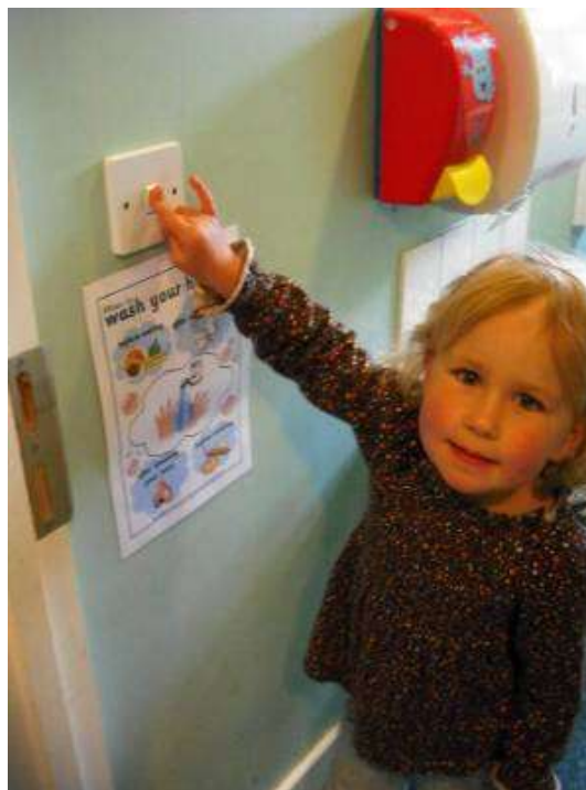
Light monitor switching off the toilet light
