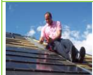
PV roof tiles (Source: JoJu Ltd)
